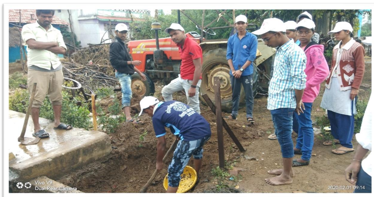
The NSS volunteers digging the absorption pit at adopted village, Gandhinagar
