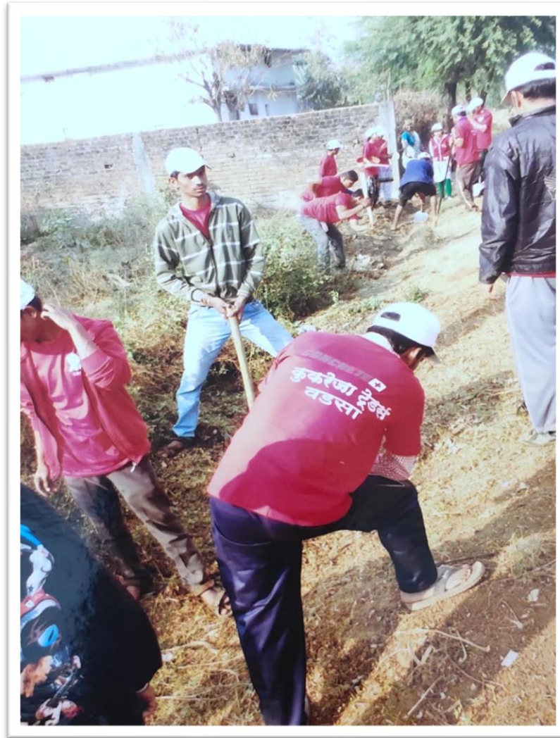
Students Constructing new canal at adopted village through labour donation
