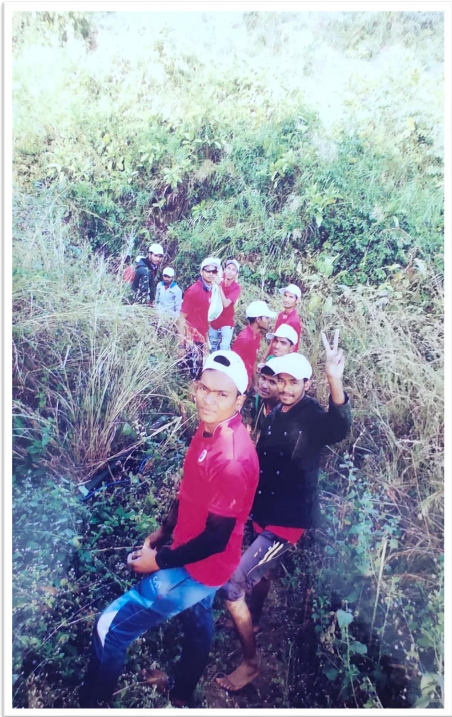
Students Constructing barrage through labour donation
