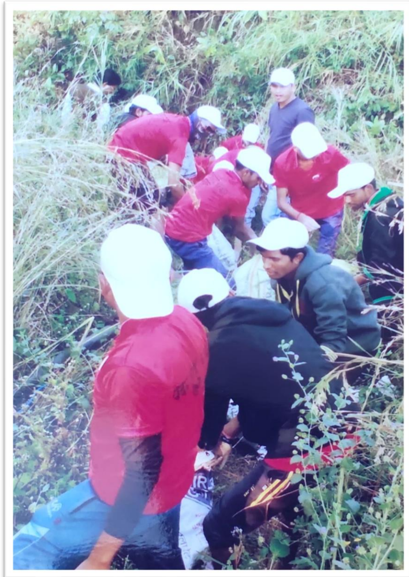
Students Constructing barrage through labour donation
